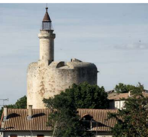
Aigues-Mortes Towers and Ramparts
