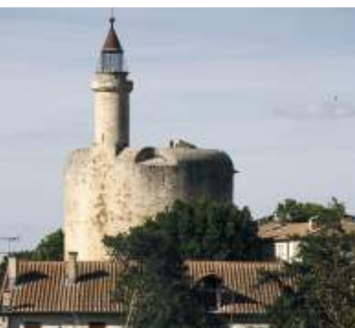
Aigues-Mortes Towers and Ramparts
